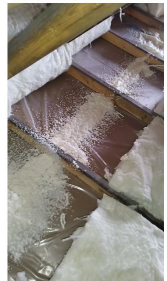
Air sealing penetrations into the attic space
