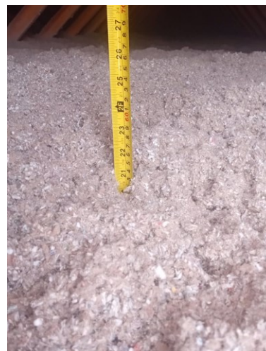
Final insulation levels
