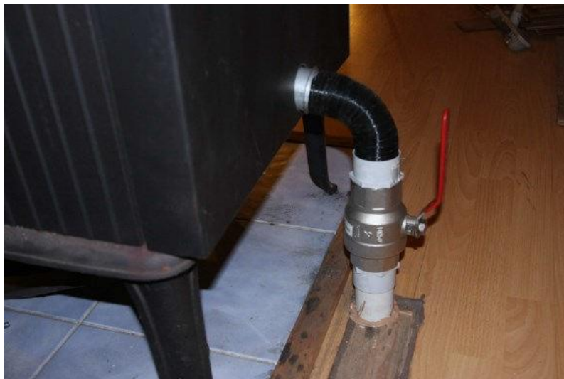
Direct venting of a wood stove with a pipe through the floor and a valve
