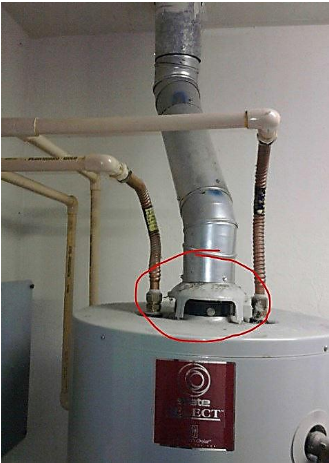
An open draft hood at the top of a hot-water tank circled in red
