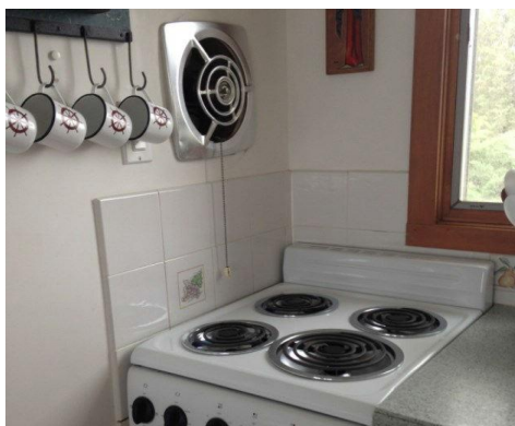
A basic exhaust fan over a stove
