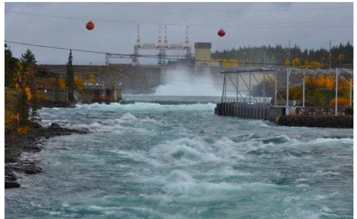
The hydroelectric generation dam in Whitehorse, Yukon
