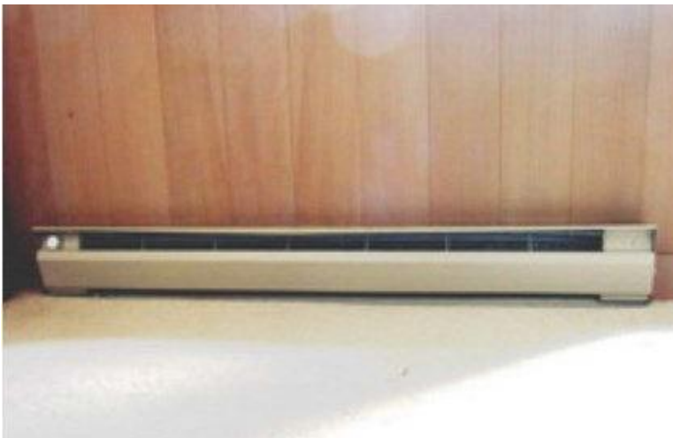
A typical electric baseboard heater that would be located in each room of a house
