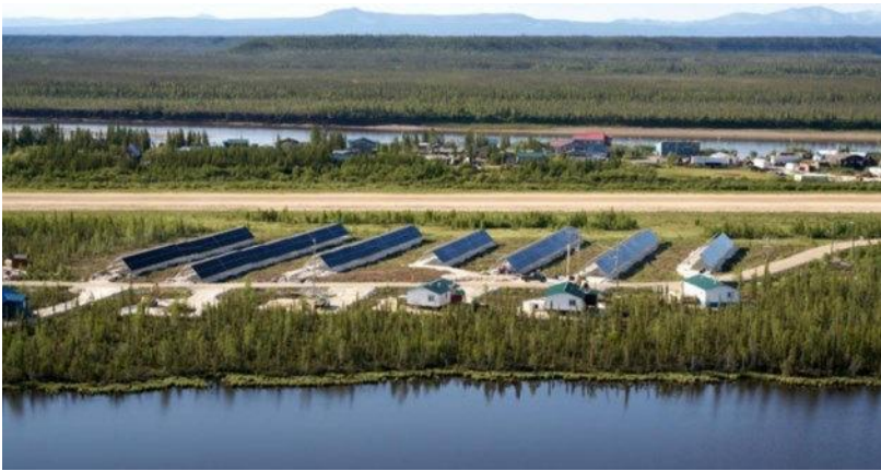
Solar farm installation
