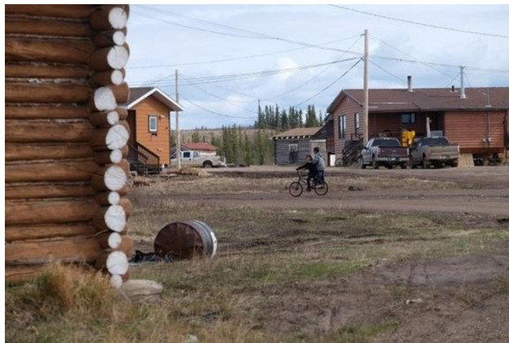
Power-pole installations in a community
