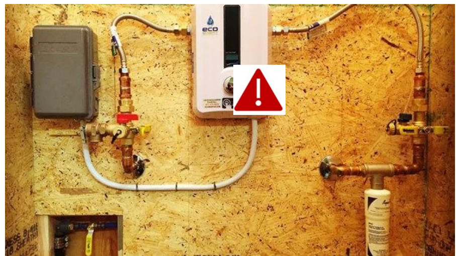
Instantaneous hot-water heater
