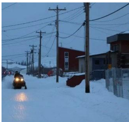
Power-pole distribution in a community
