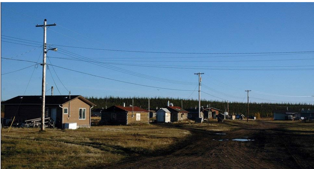
Power-pole installations within a community
