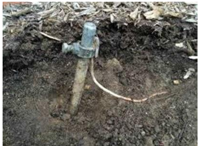
Typical ground installation
