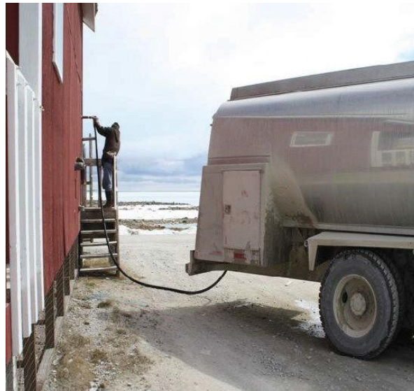
Worker filling up a house's water tank at the fill port with a hose from the water delivery truck
