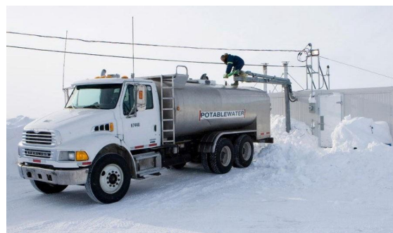
A water truck being filled at a water treatment plant's fill station
