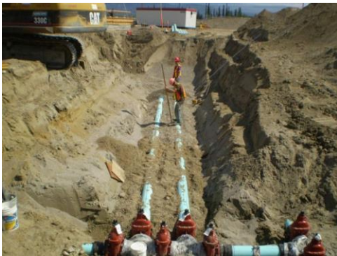
Water supply pipes being installed in a trench
