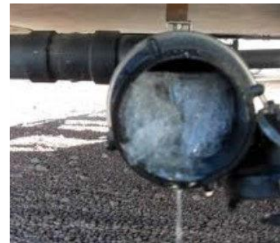
A frozen pipe filled with ice
