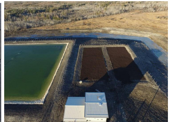
A sewage lagoon with multiple ponds
