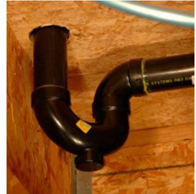
A typical plumbing trap in a house
