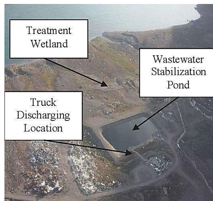
A sewage lagoon with a single pond that flows into a wetland
