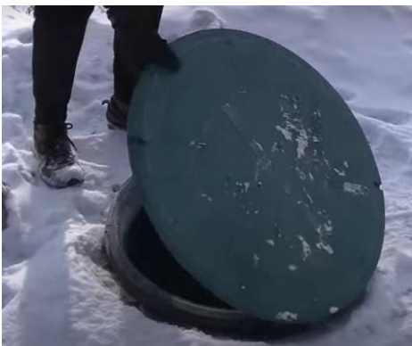
Opening the cover of a septic tank to break up the ice in the septic tank
