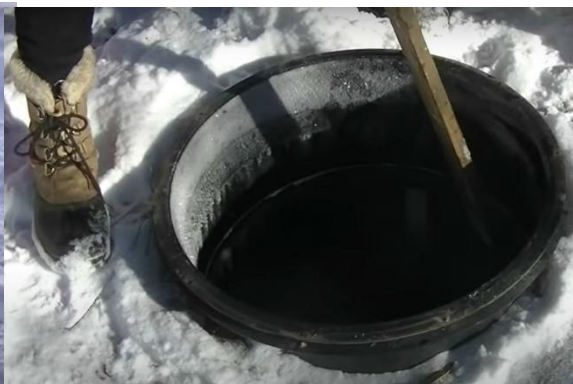
Opening the cover of a septic tank to break up the ice in the septic tank
